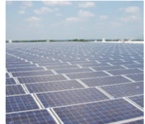
Seagull Lighting (Riverside, NJ)
